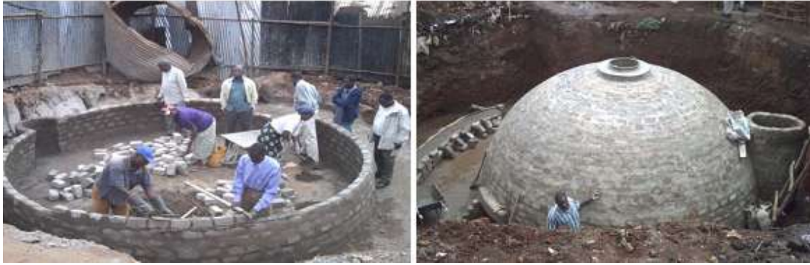
Figure 4 a - b: Construction process of the bio-centre
