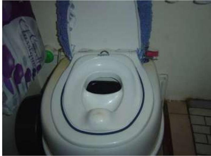
**Figure 4: A UDD toilet with a kiddie seat in Hull Street (Source: CSIR, 2011).**
