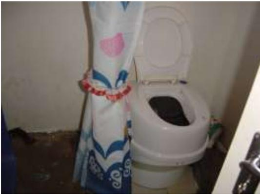
**Figure 8: Indoor UDD toilet in Hull Street (Source: CSIR, 2011).**
