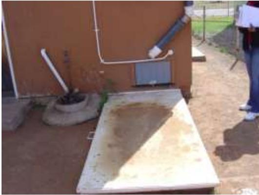
**Figure 10: Door to access a faecal vault from outside the housing unit (Source: CSIR, 2011).**
