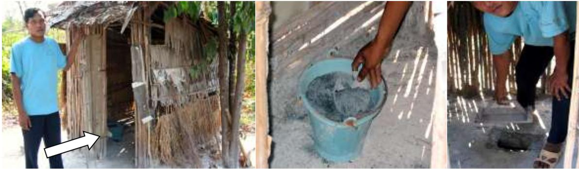
**Figure 15. This startling innovation of using ash in dry pit latrine and covering the pit with a fly proof lid by a farmer in Skun village, Banteay Srei, Cambodia, the 1<sup>st</sup> ODF village has been spreading not only in Cambodia but in many countries in Asia and Africa. Watch the bucket full of ash kept inside.**
