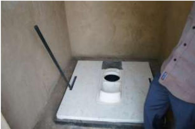
Figure 8. Inside of the pilot model for squatting type toilet
