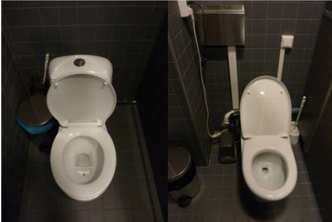
Figure 5. An Eco-Flush urine-diverting and water-saving toilet (left) and a Jets vacuum toilet seat with its pump (right).
