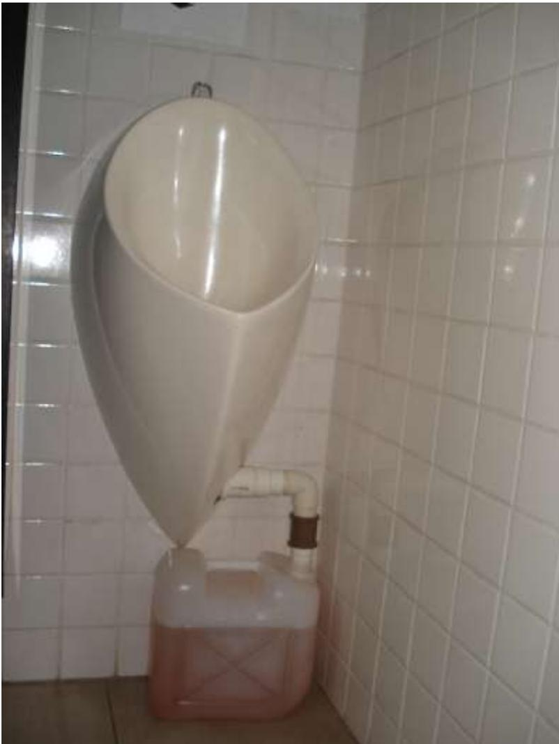
Figure 1- Waterless urinal installed in a male toilet in the *campus*.
