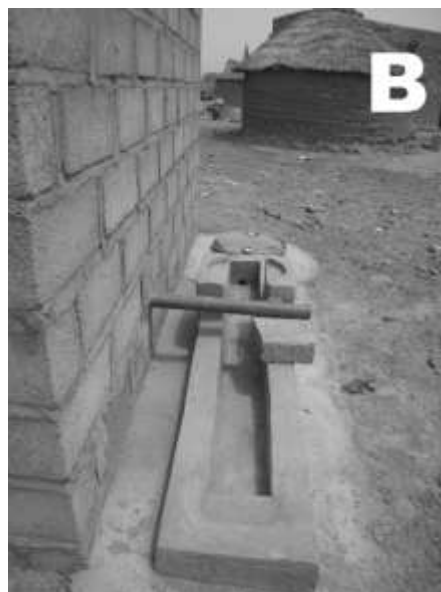
Fig. 2 Composting toilet (A) and slanted soil system for greywater treatment (B)
