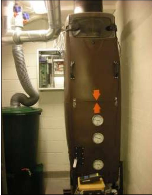
Picture 1. Dual-layer dry toilet composter (right) with Naturum urine tank (left) and gas control system (back)
