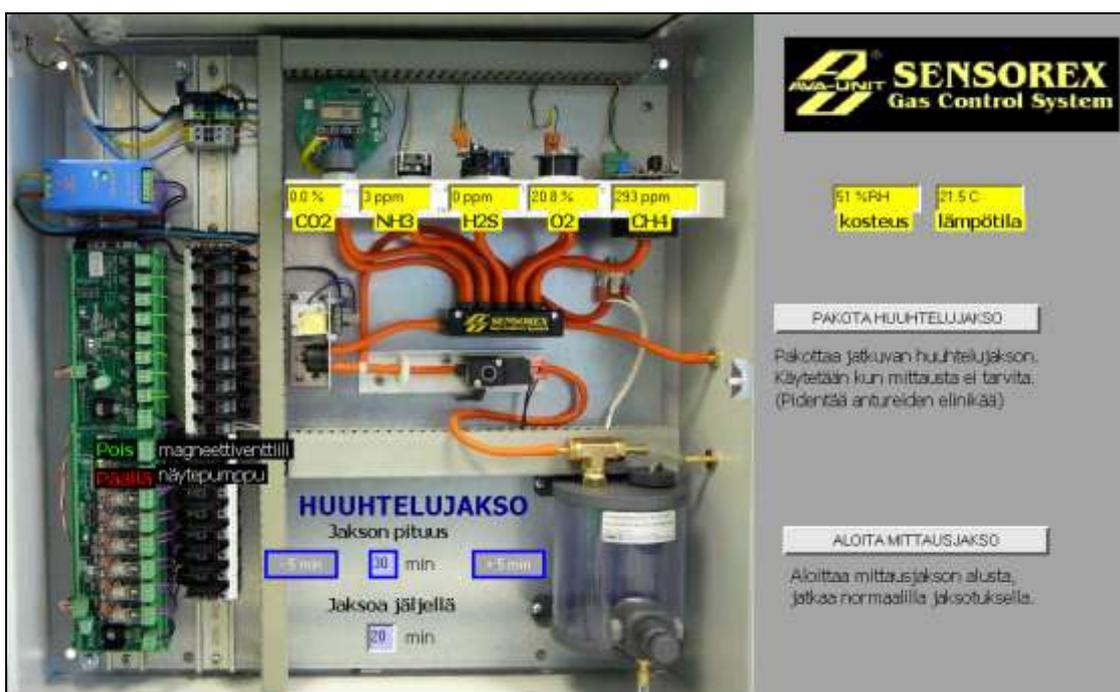
Picture 3. Control panel of Sensorex gas control system
