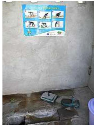
**Figure 1.** View inside a UDDT cubicle, at Kendu Muslim Secondary School with an explanatory poster on the wall, squatting pan with urinating hole and two holes for faeces leading to two vaults that are used alternately. In the right corner is a bucket for ash as dehydration material. The lids for the two faeces holes are also visible.
