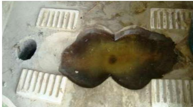
Figure 2 Urine pipe blocked at intervention area, Surkhnet.
