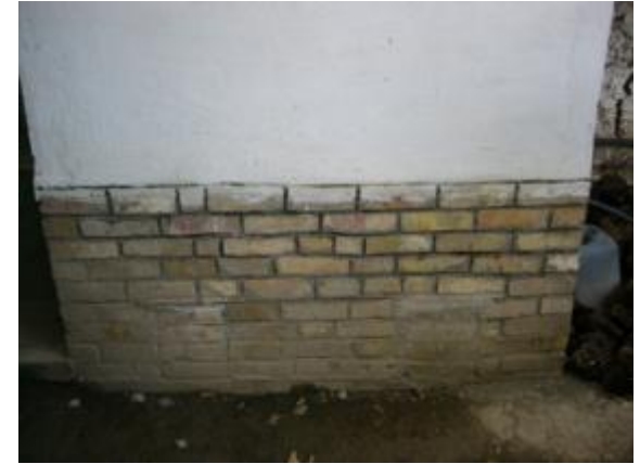
Closed with bricks and mortar
