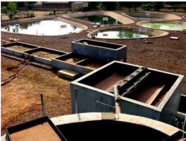
2iE wastewater treatment plant
